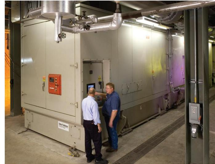
*15 MW gas turbine generator set at Michigan State Univ., Solar Turbines Inc.*
