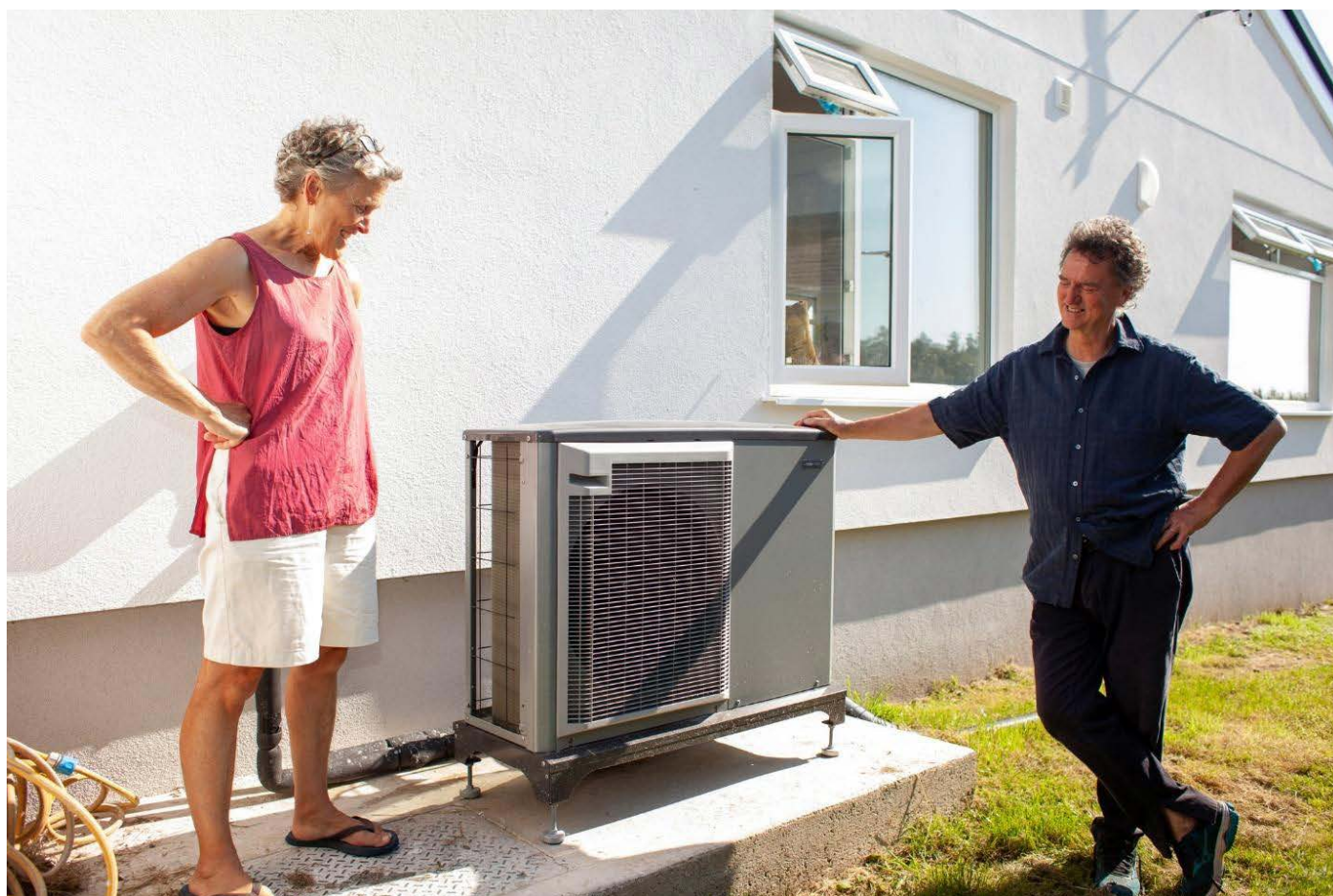
A domestic air source heat pump. Image kindly provided by Jonathan Atkinson AKA @lowwintersun.
