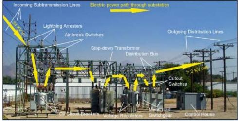
Figure 1. Energy flow through a typical substation
