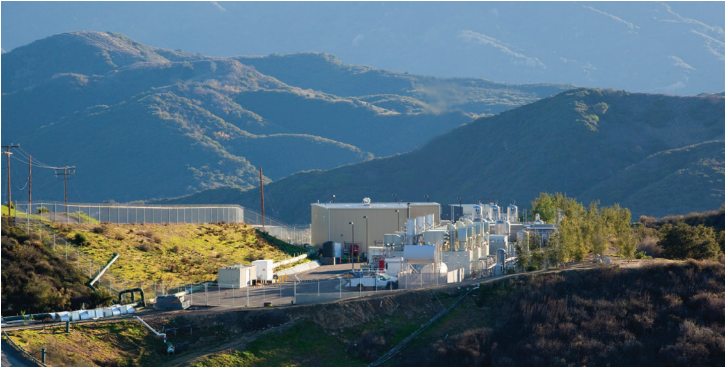
Three 4.7 MW Mercury™ 50 recuperated gas turbine generator sets are at work at this landfill gas to energy facility in Agoura, California. Photo courtesy of Solar Turbines Incorporated.
