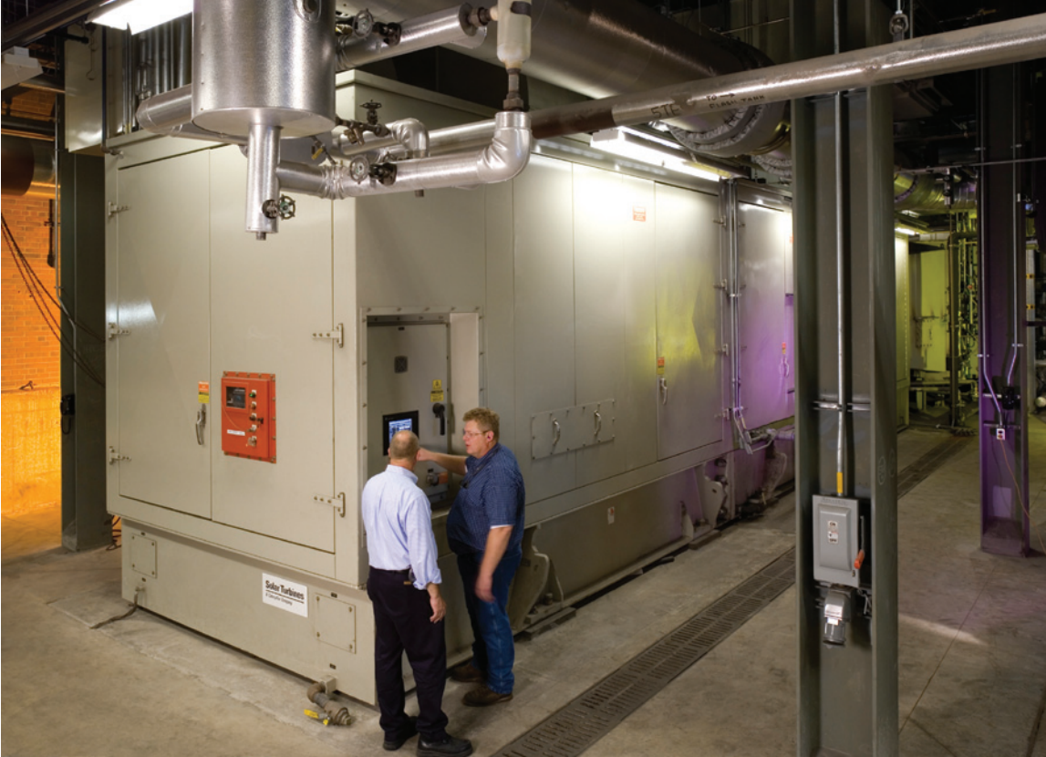
One 15 MW Titan™ 130 SoLoNOx™ gas turbine generator set provides electricity and steam for this campus at Michigan State University. Photo courtesy of Solar Turbines Incorporated.
