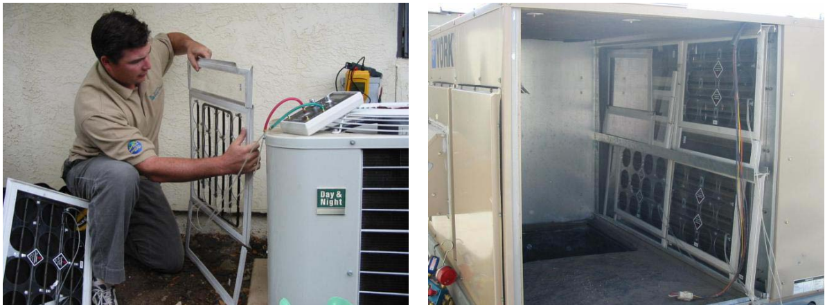
Figure 7.10: Airflow Measurements Using a Flow Grid
